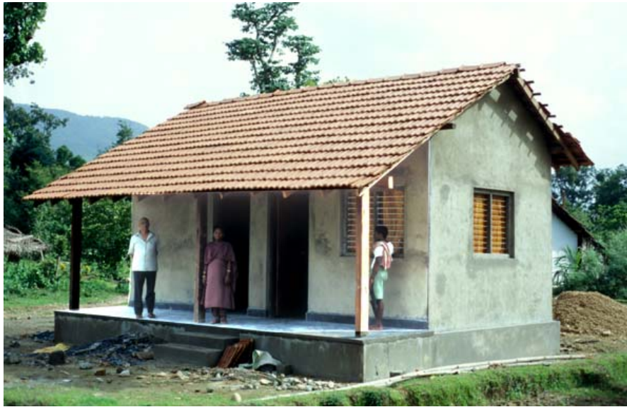
The newly constructed school building (front)
