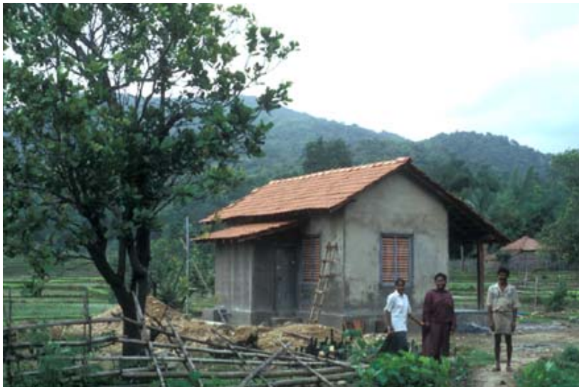
The newly constructed school building (rear)
