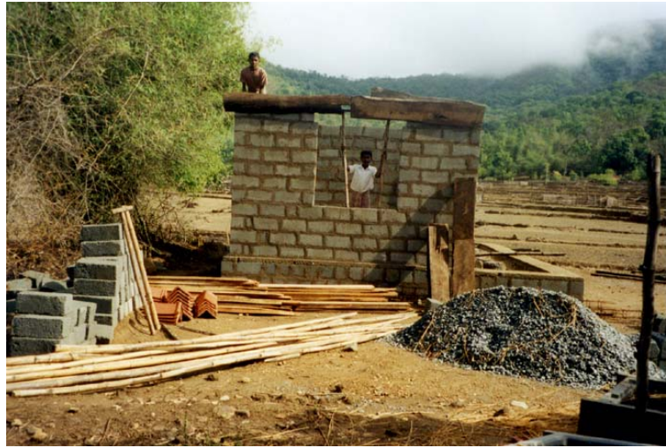
School construction with young helpers from village
